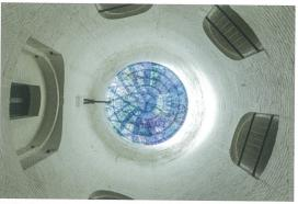
Above and left The dome consists of three parts: a wooden construction; a steel suspension system and 600 glass tiles the Glasmuseum Leerdam made together with local children.
